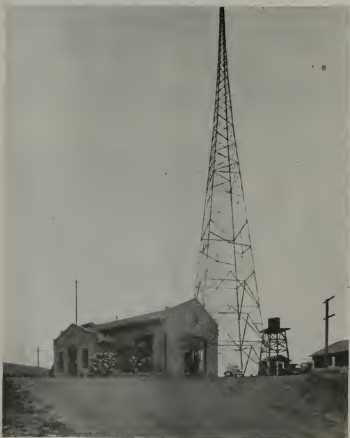
Close up view of Mussel Rock Transmitting Station, of Globe Wireless Ltd., located 15 miles south of San Francisco. Here are housed the high powered transmitters used in transpacific communications service.
